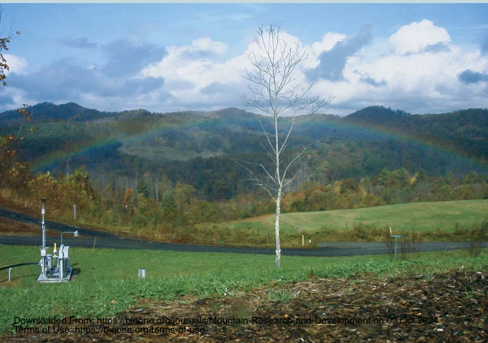
FIGURE 2 Capped landfill with methane recovery operation in Yancey County, North Carolina. (Photo courtesy of Energy Xchange)
